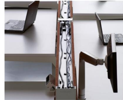
Cabling through Central cable gutter (on top)
