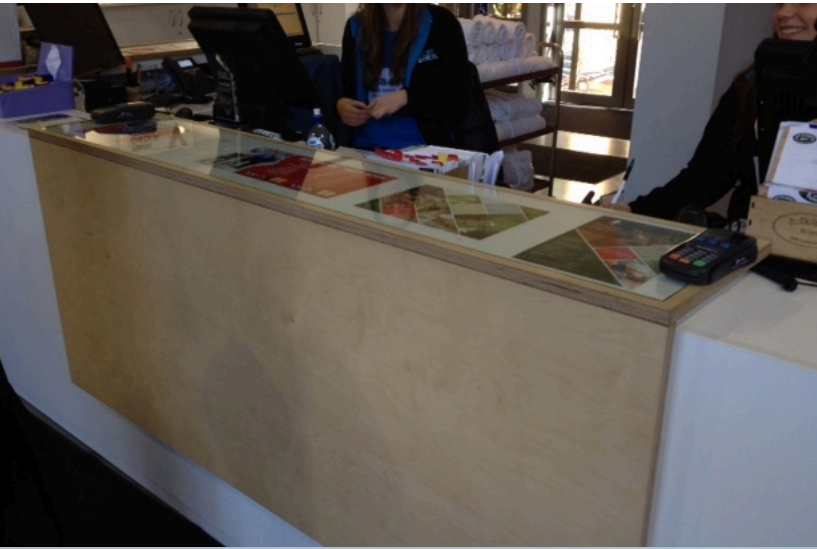
Custom made Reception counter with Ply feature panels, LED strip lighting and Glass inserts on top of feature panels for brochures.
